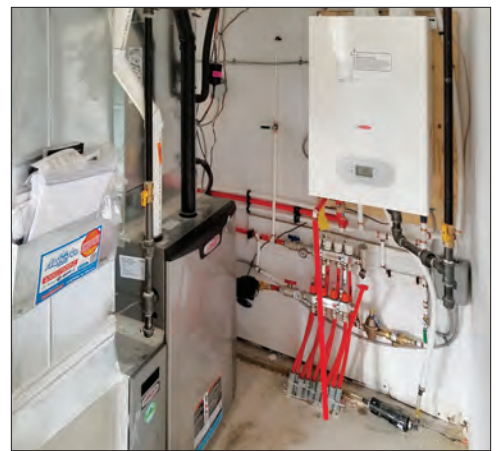
Jim Couperthwaite of Geranium Homes with newly installed Greyter HOME system. Upper right: Typical Model slab on grade design due to high water table. Right: Two-stage furnace with tankless hot water heater for radiant floor and domestic hot water.
