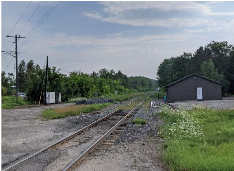
Photo 6 – View of railway line west of Site, facing east.
